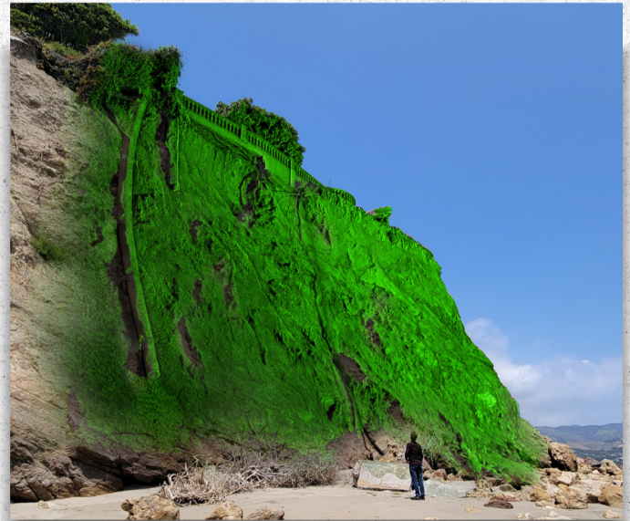
3D Laser Scan - Cliffside Erosion
