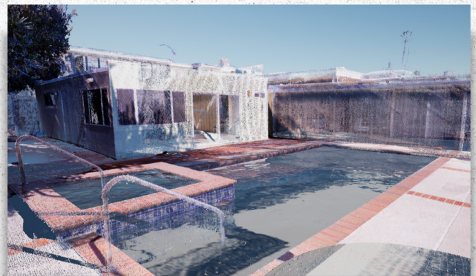
3D Laser Scan - Apartment Complex
